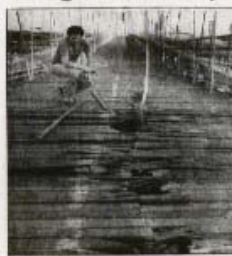
Newman checks walkway holes after two cables broke.
